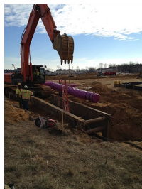
St. Charles construction site Source: CPV
